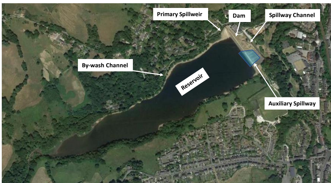
Figure 1. Location of the dam and its Principal Features
