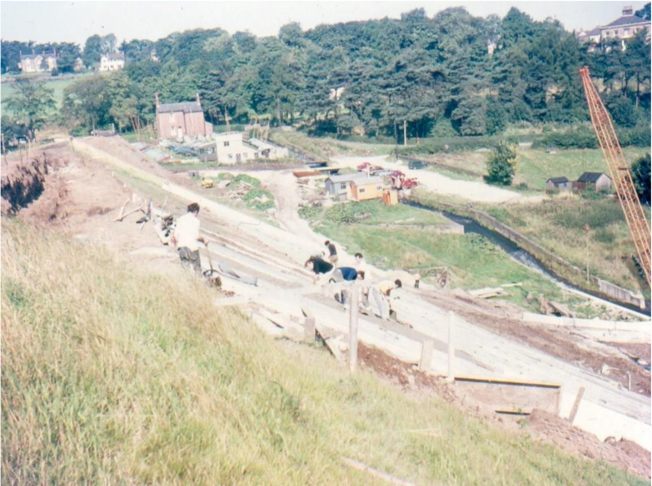
Figure 3. Construction of the Auxiliary Spillway on the Earth Embankment Dam in 1969
