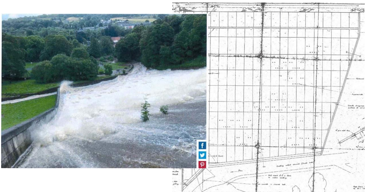
Figure. B7 Plan of the auxiliary chute and photo of flows impacting against the oblique left side wall
