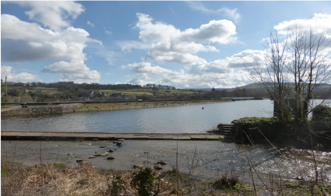
Photo GA1. The very shallow Convergence Basin viewed from Reservoir Road showing the upper end of the primary weir with a drop into the Basin of only 4 in. overall. The Bypass flow here is about 2 in. deep. A large mud bank is in the foreground taking up valuable capacity..
