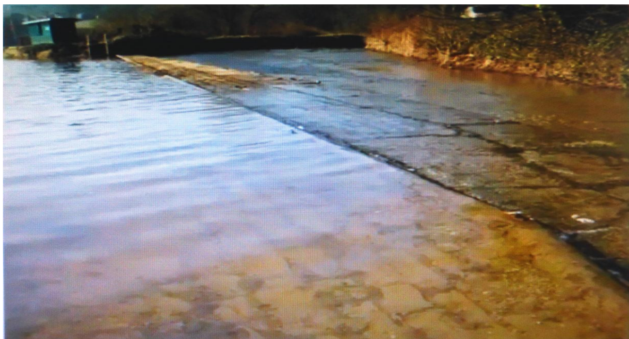
Photo 3. The view upstream showing a modest low volume overflow from the reservoir over part of the Primary Cill. ( Photo ex July Seminars )
