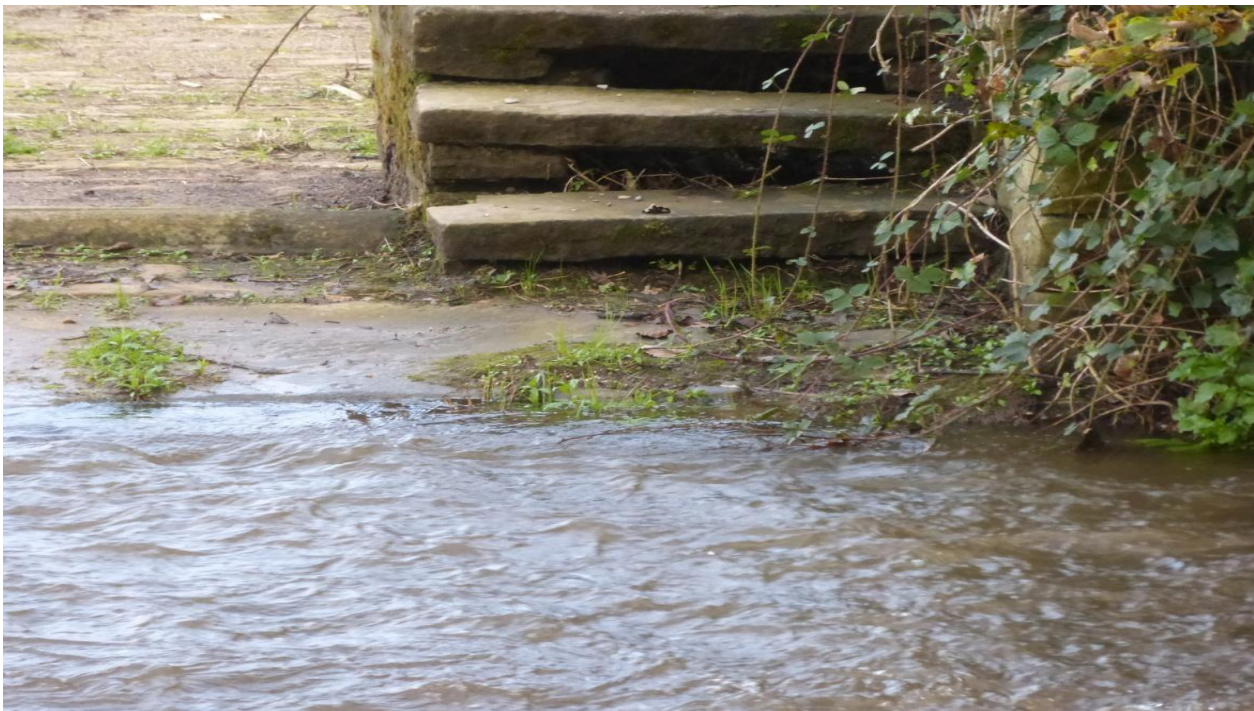
Photo GA2. Here the Bypass flow has risen, now full to the brim at about 4 in. deep, flowing to the left. If it rises by another 3 in. it will flow over the Primary Cill 'backwards' to fill the reservoir !
