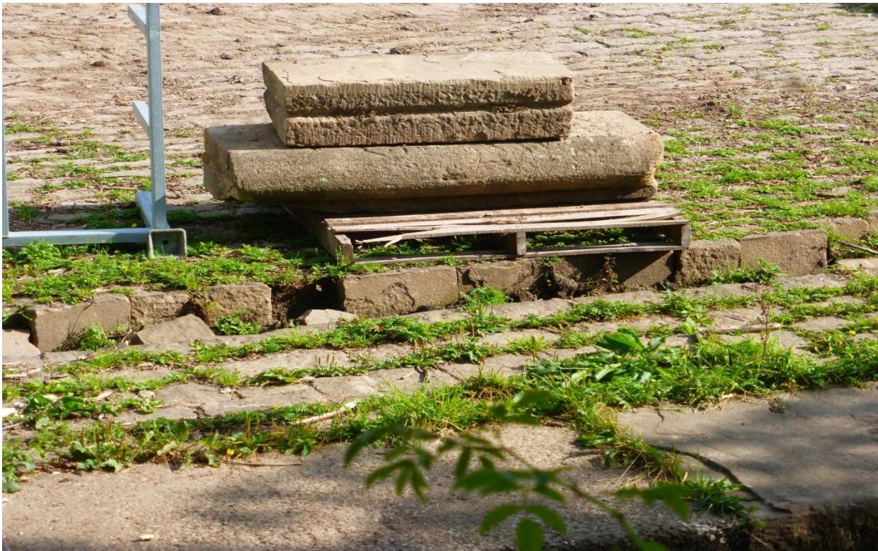
Photo 7. The Weir Blocks of the Primary Cill.
