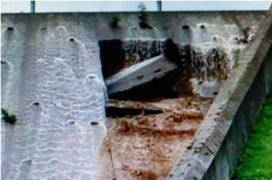
Photo 9 (above): Spillway below Gaps 1 & 2. It was probably taken late on 1 Aug., after 36 hours of the massive flow. Here the water is still over flowing, the first panels have snapped and collapsed into the deep hole caused initially by water flowing underneath the Apron.
