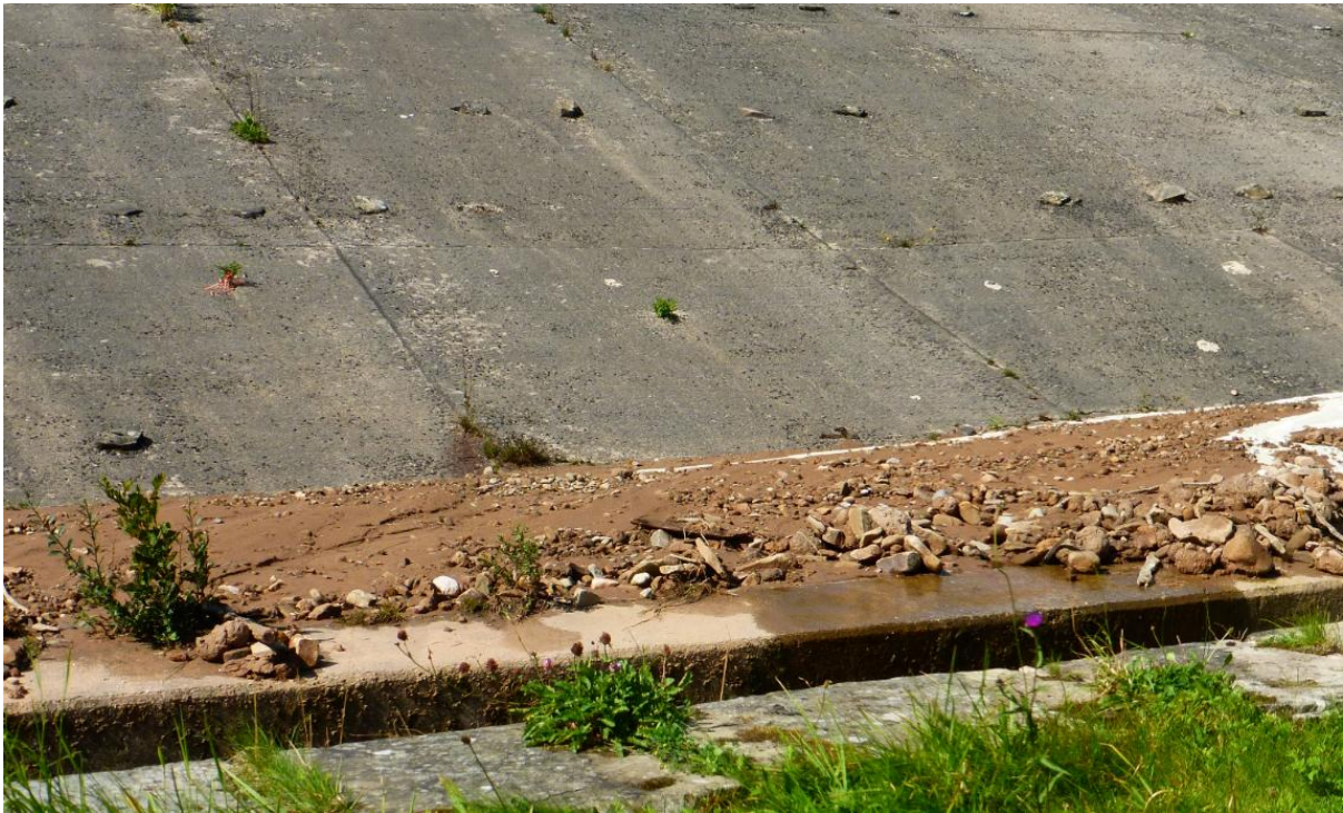
Photo 17 above & 17a. Some of the clay core on the foot of the spillway, the rest went into the Bypass and then on to the River Goyt.
