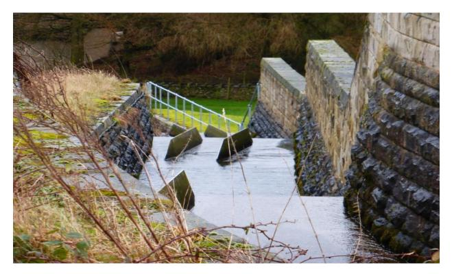
The Horse Coppice Reservoir Bypass Guide Blades. Ten blades steer the flow to avoid damage and high loads on the LH wall, exactly as is required at the Toddbrook Bypass Bend.
